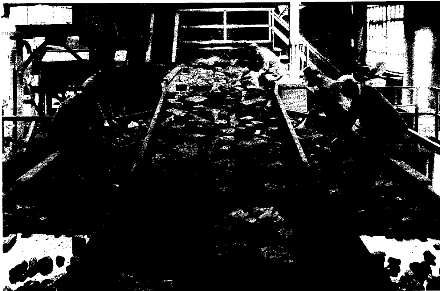
"Bone pickers" hand cleaning coal at the Virginia Iron, Coal & Coke tipple, Tom's Creek, Virginia, 1931. Such labor-intensive cleaning methods were gradually replaced by crushing, shaking and washing equipment. N&W Railway Archival Collection - VPI&SU Libraries (Blacksburg).
